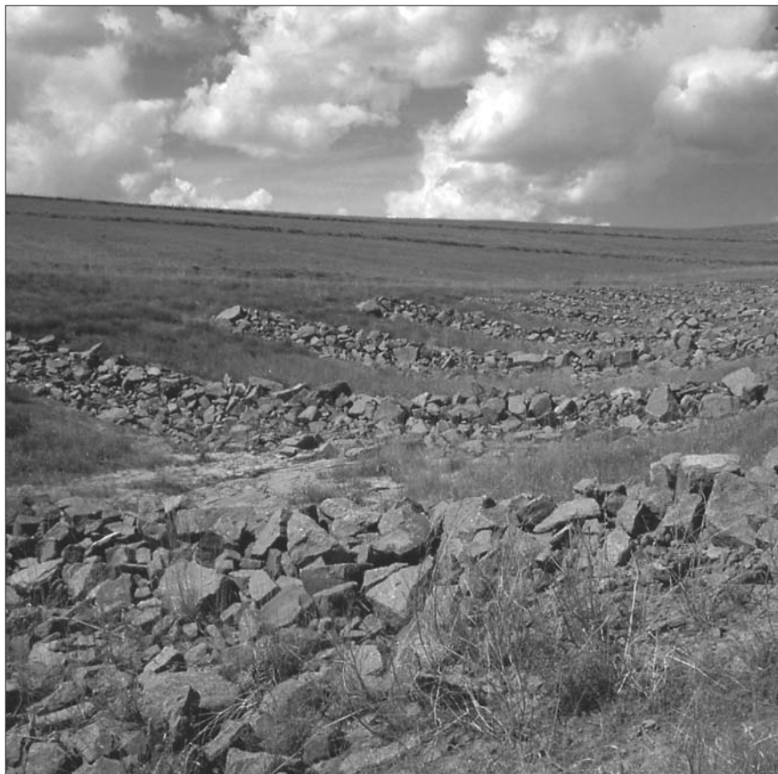
The Shirley Basin Project, located south of Casper, Wyoming, reclaimed five large abandoned open pit uranium mines. Mining operations that began in 1959 left about seven-and-a-half square miles of land containing large water-filled pits, and over 72 million cubic yards of mine waste, much of it contaminated with radioactive materials. Over three miles of the Little Medicine Bow River was rerouted, returning the river to its original drainage pattern. Almost six miles of highwall were eliminated and stabilized, 37 miles of erosion control diversions were constructed, and over eight miles of ephemeral stream channels were reconstructed. At a cost of $30 million dollars, this was one of the largest reclamation projects in the country to be funded by the Abandoned Mine Reclamation Fund. Eight years of work have eliminated the hazards and created a valuable recreation area and wildlife habitat.
