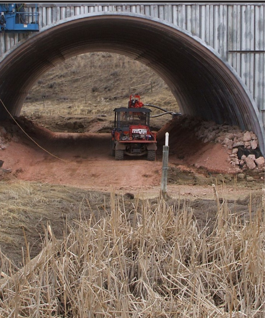
Crews construct an arch for water and wildlife to pass through at Western Fuels' reclaimed site in Wyoming.
