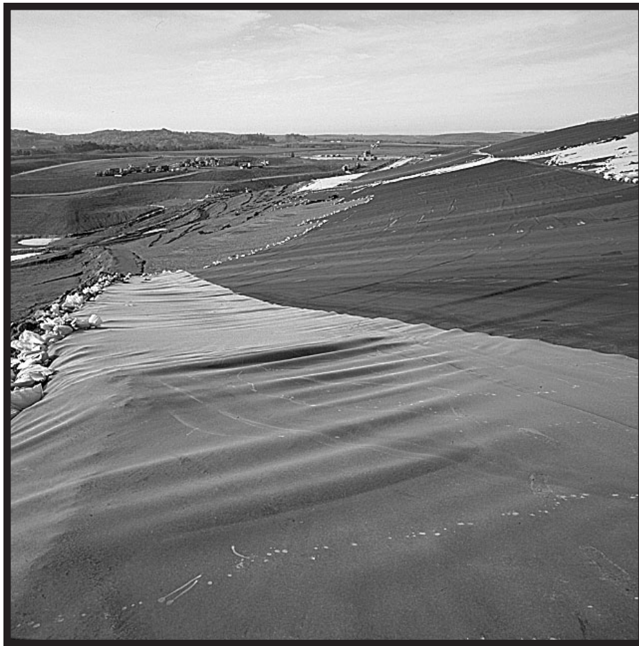
Heavy plastic liners were spread over this graded mine site near Pittsburgh, Pennsylvania to create a pollution barrier for a large landfill. Reclamation for this land use required careful grading to provide even slopes and a clean surface. Multiple barriers of plastic and soil prevent leakage and provide drainage to the bottom of the fill for collection and treatment. In the future, the entire valley of this former mine will be filled with refuse and covered with earth.
