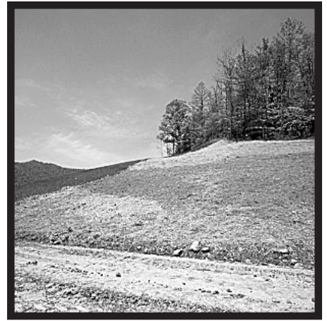
As overburden and coal are removed highwalls are formed. Highwalls can be more than 100 feet high and extend thousands of feet. One of the most widespread and dramatically visual problems prior to the Surface Mining Law was highwalls that were left exposed when a mining operation was completed. This regraded and mulched slope at a mining operation in Pike County, Kentucky (above) has been blended with the surrounding terrain and is typical of reclamation under the Surface Mining Law.
