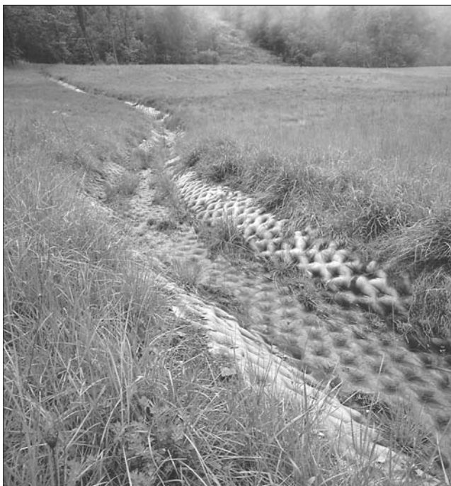
At this West Virginia abandoned mine reclamation site a concrete lined channel was used to prevent erosion. This quickly installed structure allowed drainage from the steep woodlands above the project to run down the reclaimed slope without causing damage. In a few years both woody and herbaceous vegetation will grow through holes in the concrete
