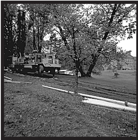
Surface subsidence resulted when the roof collapsed in an abandoned underground mine 150 feet below a residential area adjacent to a high school in Fairmont, West Virginia. After drilling 320 boreholes, 2,000 cubic yards of concrete was pumped into the boreholes. The resulting concrete pillars support the mine's roof and will prevent future subsidence.
