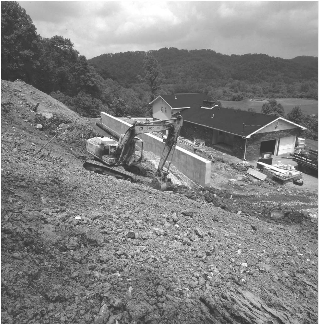
A landslide above this Kentucky house required emergency work to prevent further damage. Surface and subsurface drains at the top of the hill divert water around the house. The concrete wall will provide a solid base at the bottom of the hill and prevent future sliding. The large pipe covered with gravel behind the wall will prevent water buildup and keep added pressure off the wall. As the last step in the reclamation process, the entire site will be graded and revegetated. On September 30, 2004, there were more than 1,500 acres of dangerous slides that needed reclamation in Kentucky.
