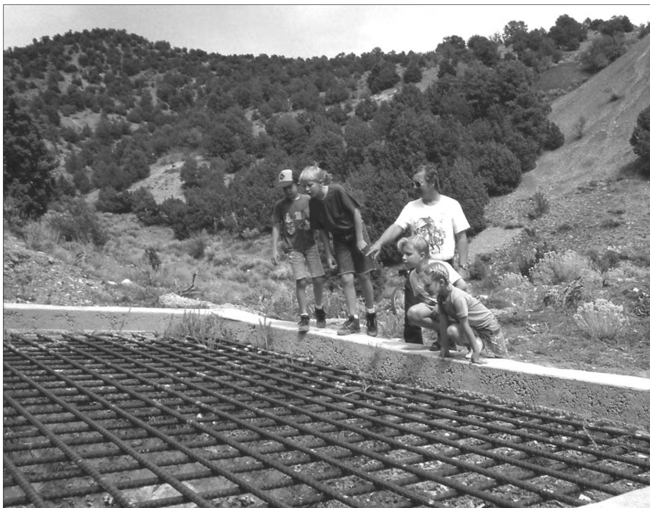
Near the town of Eureka, Utah, the Tintic project closed 41 underground mine openings. Early 1900s hardrock mining in Utah left hundreds of abandoned mine openings. Shafts and portals were a safety hazard at the Tintic site due to its popularity with hikers and mountain bikers. Some of the openings were closed by backfilling; however, many were covered by steel grates. Due to limited fill, and the need of landowners to have future access to the mines, vandal-proof grates were designed. The grates used one-inch re-bar on 8-inch centers, with welded intersections. Reinforced concrete beams were poured around the opening to anchor the structure and complete the closure. The grates provide a low-cost method of protecting the public from very dangerous abandoned shafts that otherwise would be impossible to close. On September 30, 2004, there were more than 800 abandoned vertical shafts that needed reclamation in Utah.
